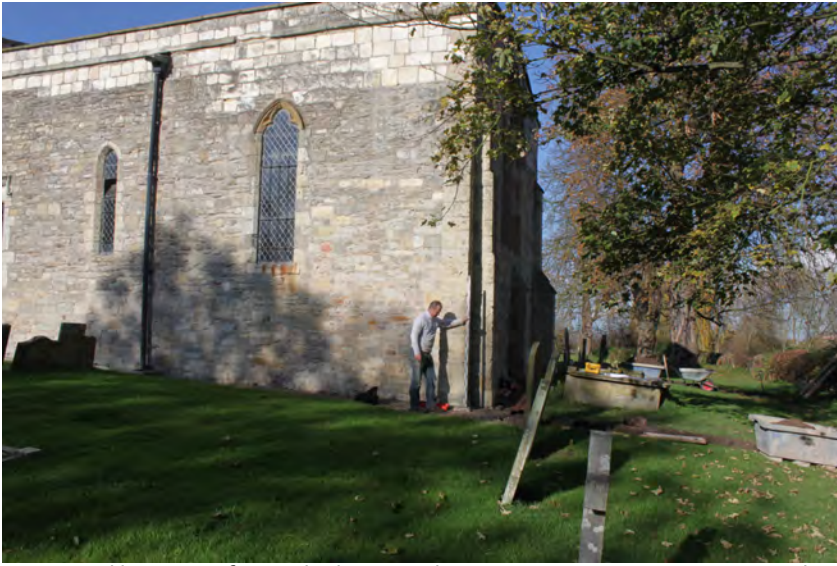
Plate 14a – general location of TBM, looking north.
