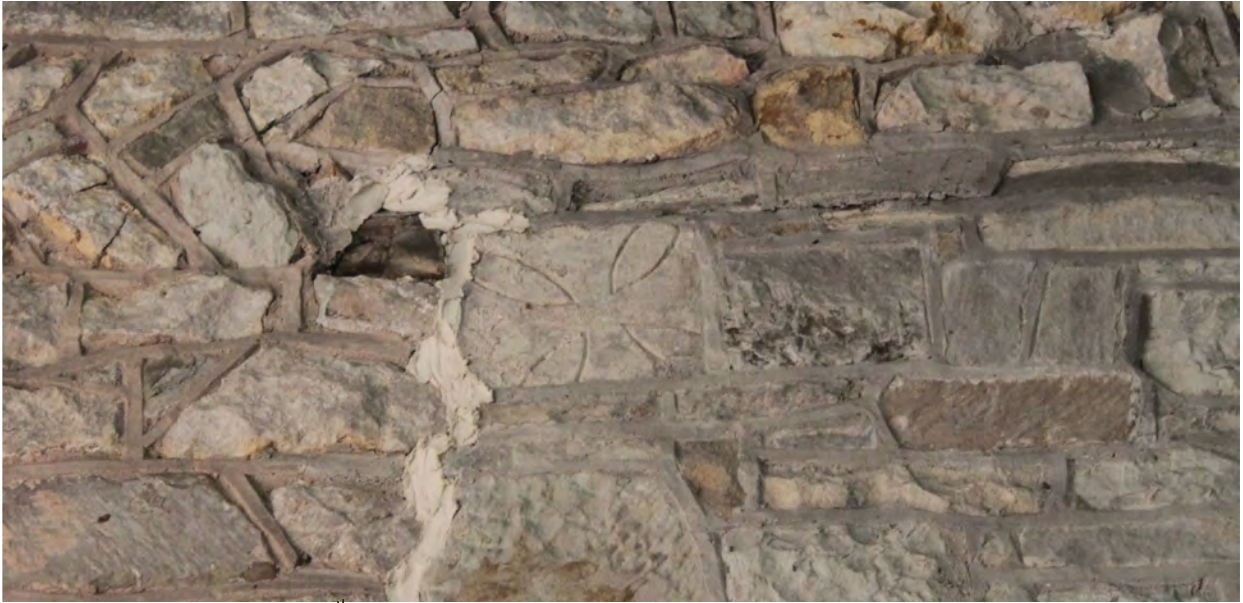
Plate 09 – fragment of probable 12 th century grave slab re-used high up in the nave wall over the south door. Looking south.
