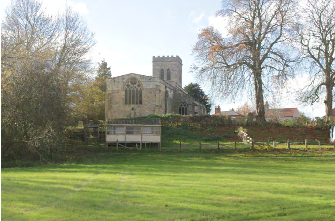
Plate 03 – St. Peter's looking west from the floodplain, with the shed in front of the church built up against the former river cliff which forms the eastern boundary of the churchyard.
