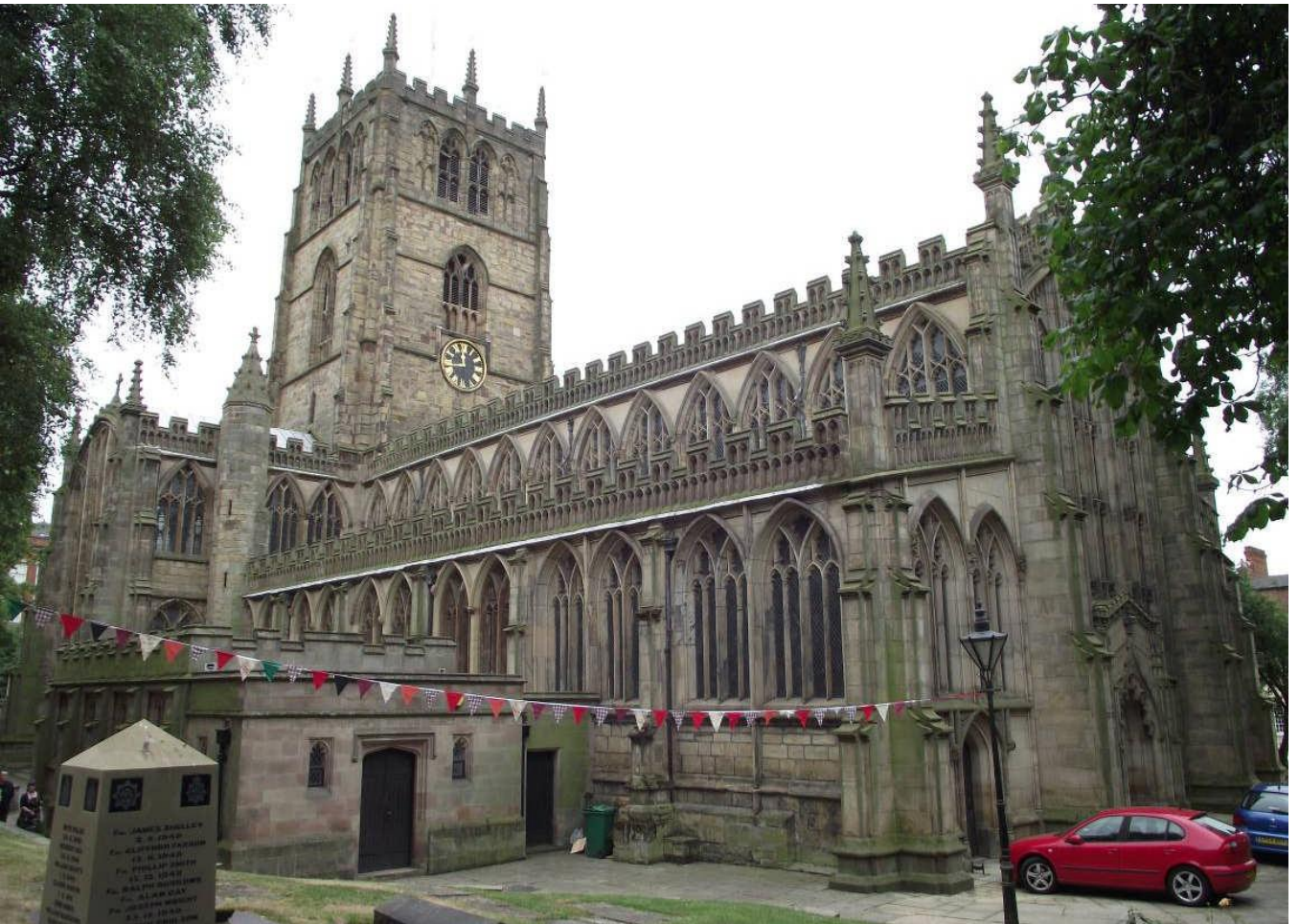
Plate 1: Church of St. Mary's from the west end, looking south-east and north-east.
