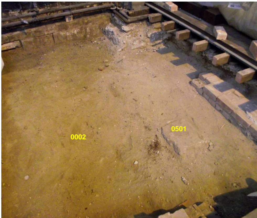
Plate 5a-b: North Transept floor during groundwork. Upper (16) looking south, bottom (15) looking south-east.
