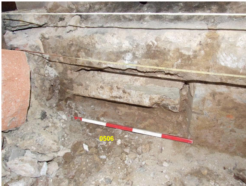
Plate 10 a-b: North Transept (15) east wall foundation 0505 (west facing) plus close up of 0506 containing window mullion.
