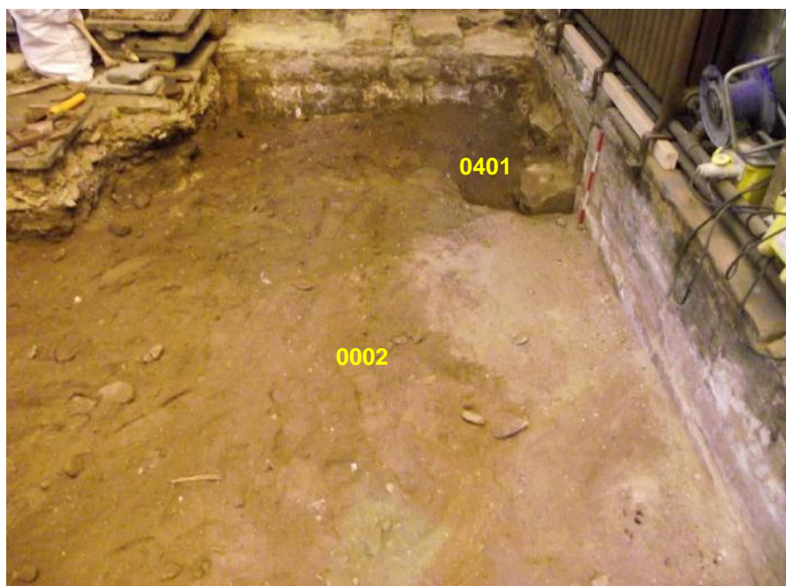
Plate 4a-c: South Transept floor during groundwork. From top looking east, middle looking south-east, bottom looking south
