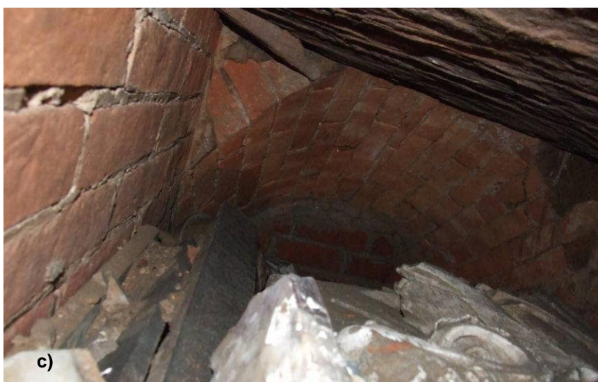
Plate 24a-c: Entrance in Plumptre Vault.
