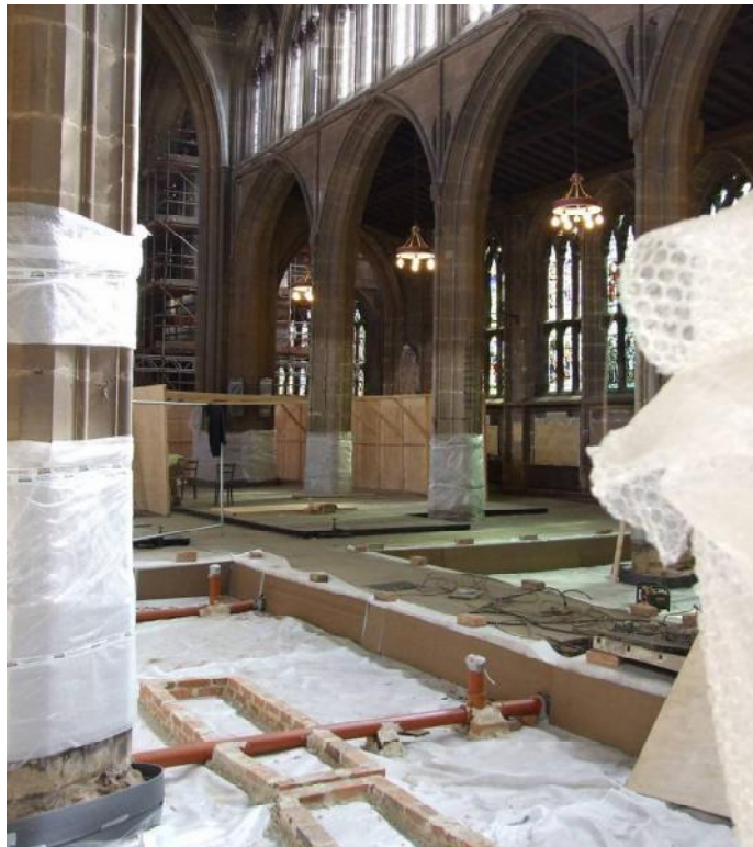
Plate 2: View of nave groundwork in progress. Upper showing removal of raised floorboards. Lower showing shallow depth of groundwork.
