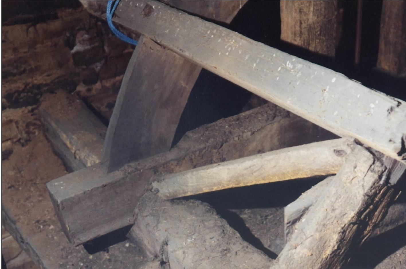
Figure 4: Later transom brace in treble pit
