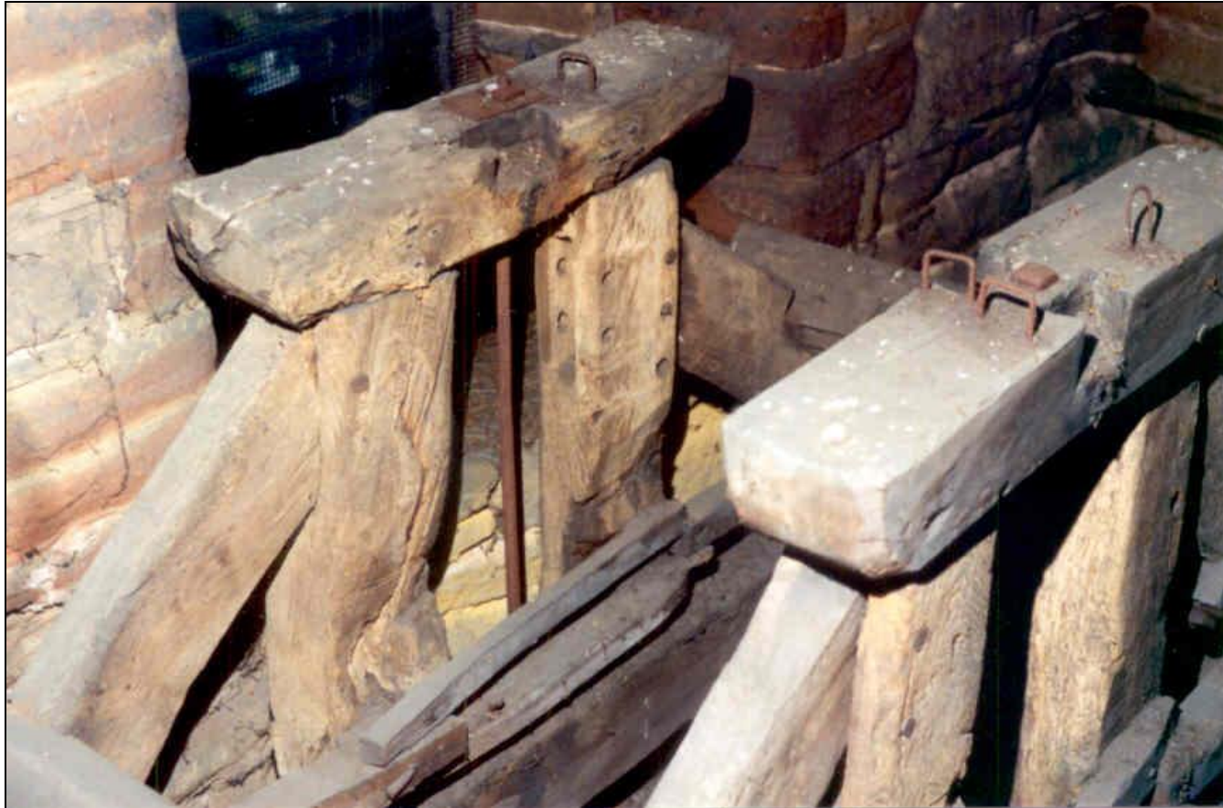
Figure 3: Truss from the treble pit
