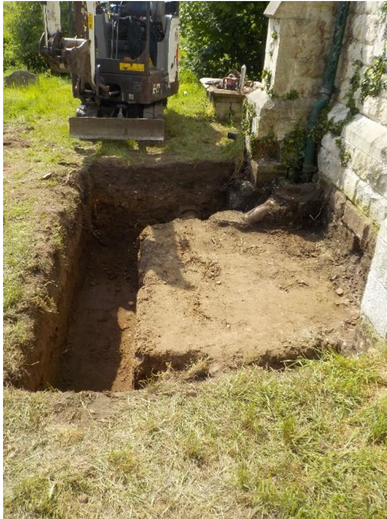
Plate 2: Extension footings (looking W)
