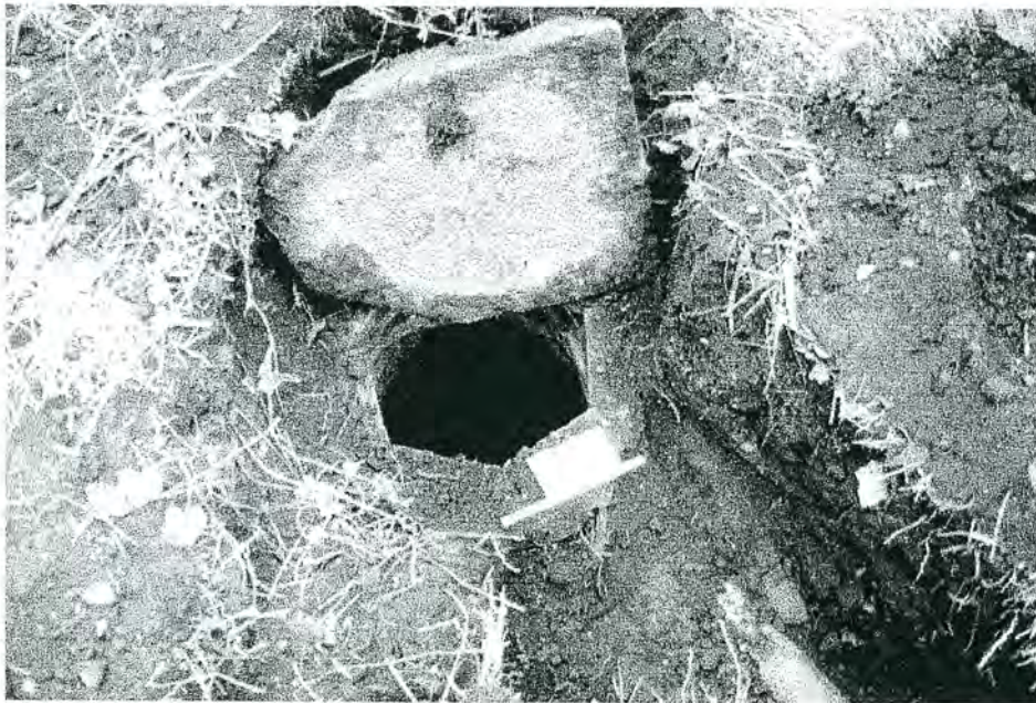
Plate 6: 01, the capstone of soakaway 0004, lifted to reveal a six-sided brick structure.
