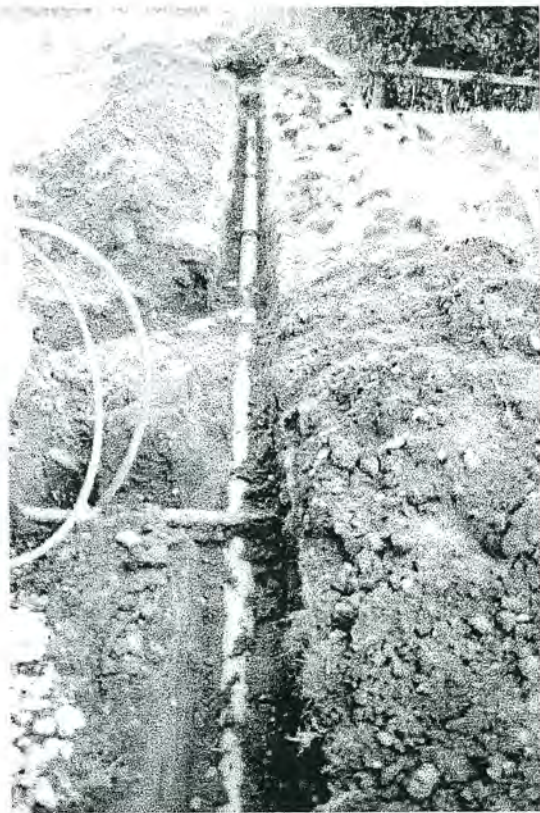
Plate 1: 01, the pipe trench running north-east of the chancel.
