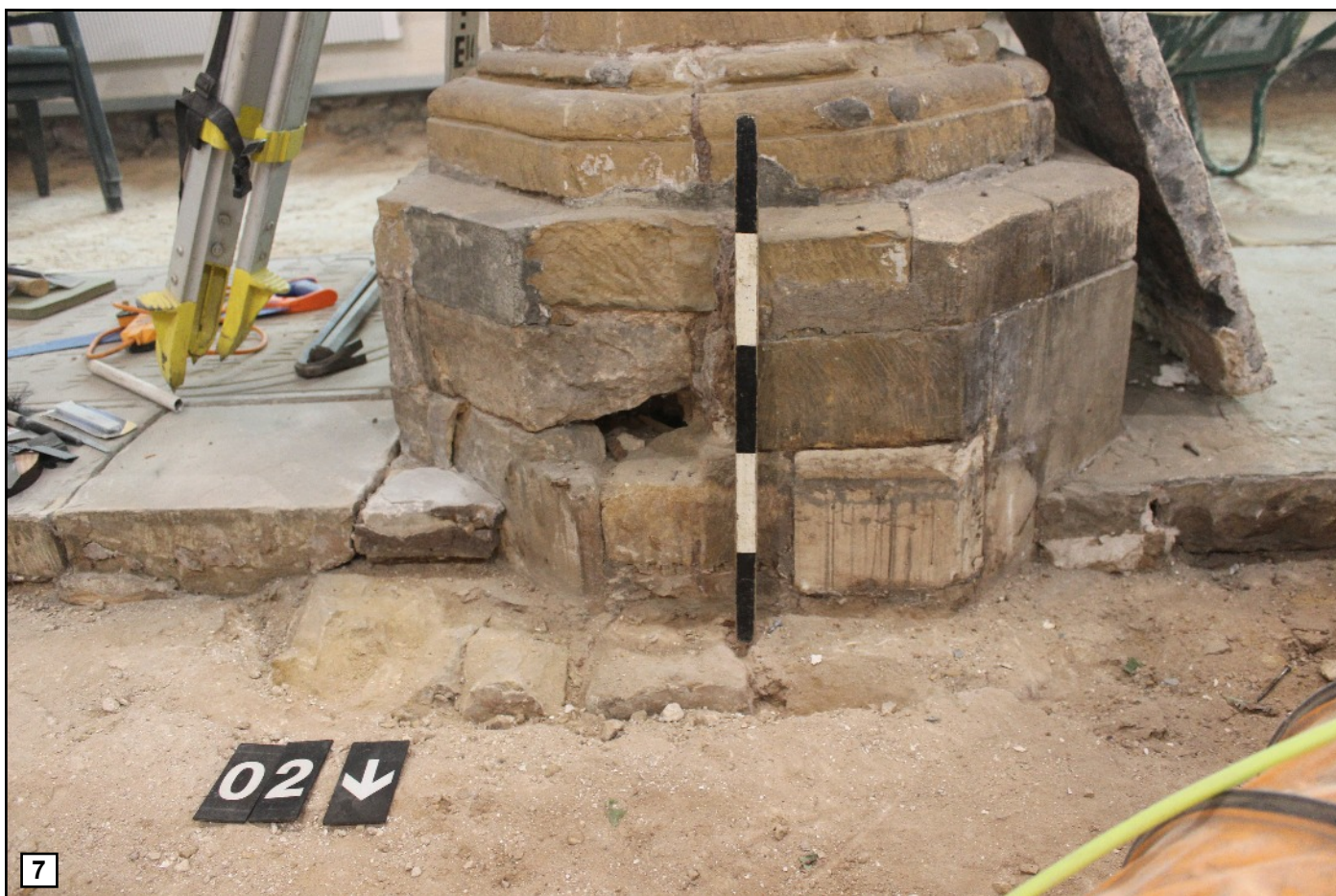
Plate 6: Western circular pier and foundation 0209 in Area 02, viewed looking north.
